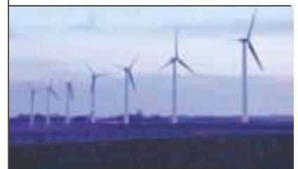
Wind farm in Wyoming.
