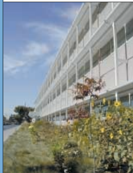
Energy efficient office building, Department of Natural Resources. (UEO)
