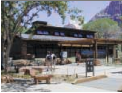
Energy efficient visitor center at Zion National Park. (UEO)
